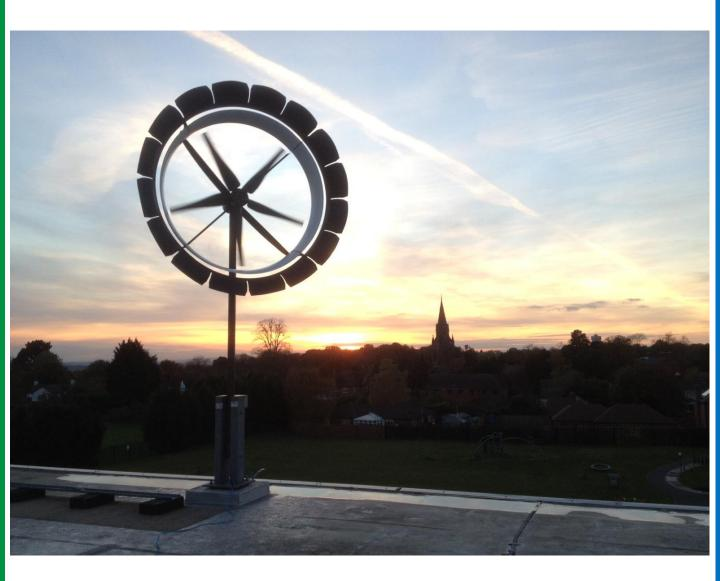
A018 with lifting pole flat roof installation
